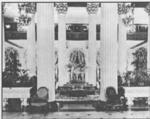
The beautiful lobby in the Champion Street entrance to the Towers.
