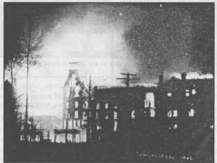
Fire destroys the San, Feb. 18, 1902.
