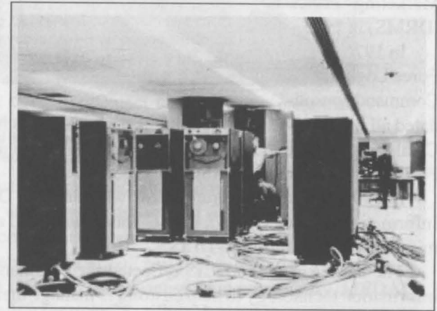
The new DLSC computer room, shown in 1977, originally held critical information necessary to all modernization efforts.
